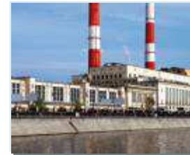
thermal power generation
