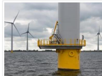
The winning consortium bid 5.45 €-ct per kWh for Borssele Offshore Wind Farm construction. (photo: iStock)
